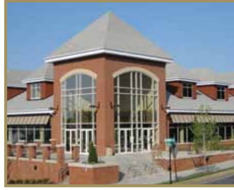
Eagle Commons dining facility, at the corner of Wood and Arnold streets, buys meat and produce from local farms when possible. The doors to Eagle Commons are open to the community, as well as to the university.
